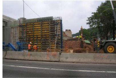
Construction of new retaining wall
