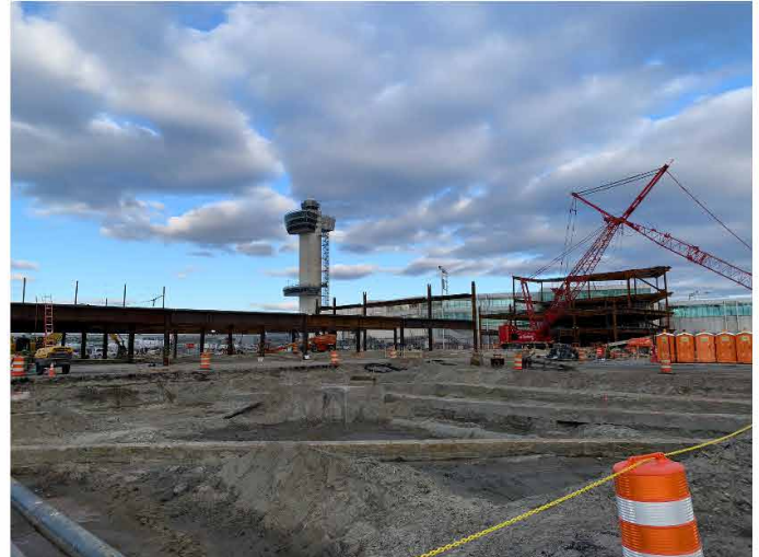
Concourse A Steel Erection
